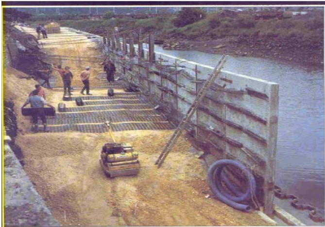
Fig 14: Laying of geogrid (Nand, K.2005).
