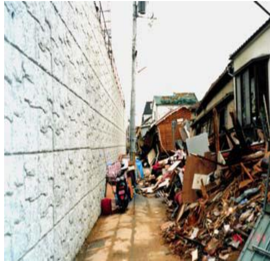
After the earthquake
