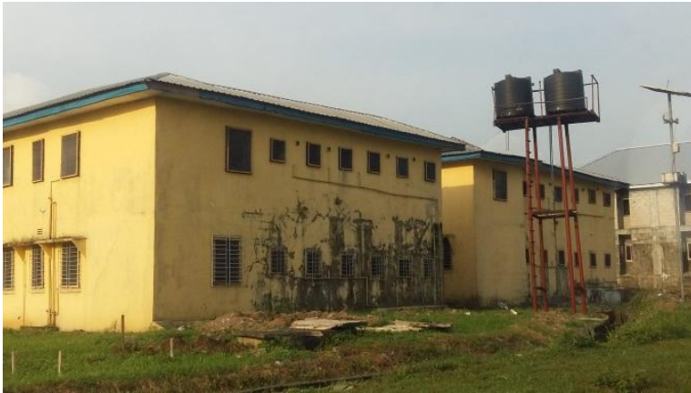
Figure 3: Showing Hostel D at R.S.U Source: Author
