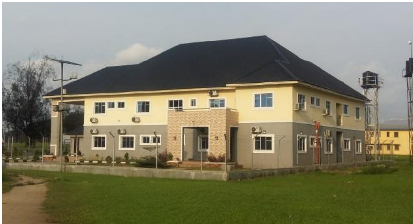
Figure 6: Showing Student Union Government building at R.S.U Source: Author
