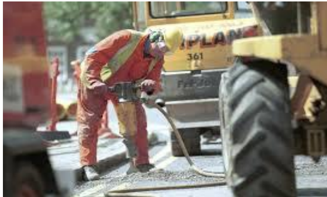
Figure 1: Construction work noise situation
