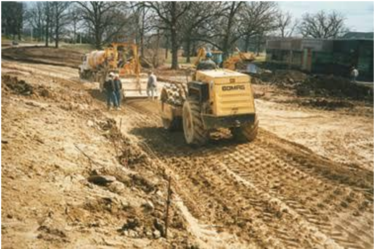
FIG. 1: An Image of Soil Stabilization Using Fly Ash ( SOURCE: U.S Department of Transport)
