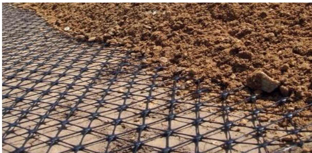
FIG. 5: Geogrid Used In Soil Stabilization (SOURCE: Geosynthetics.com)
