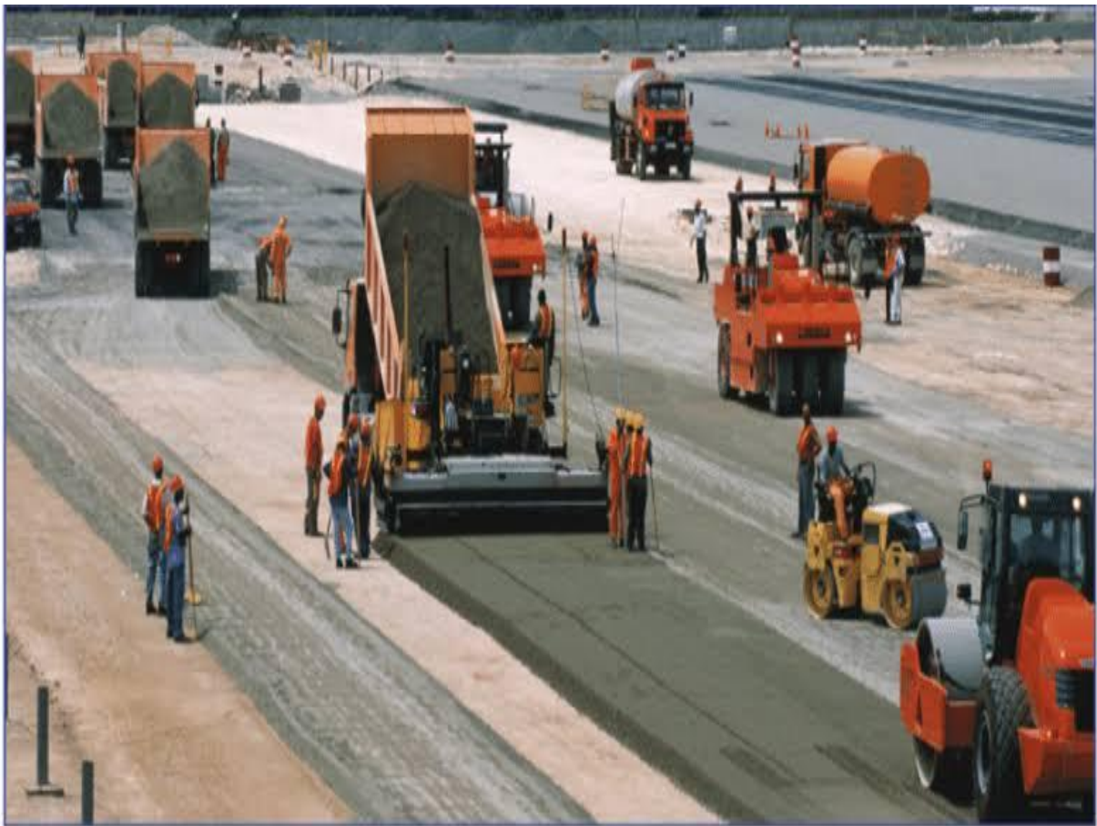
FIG. 2: Soil Cement Stabilization (SOURCE: Research Gate)
