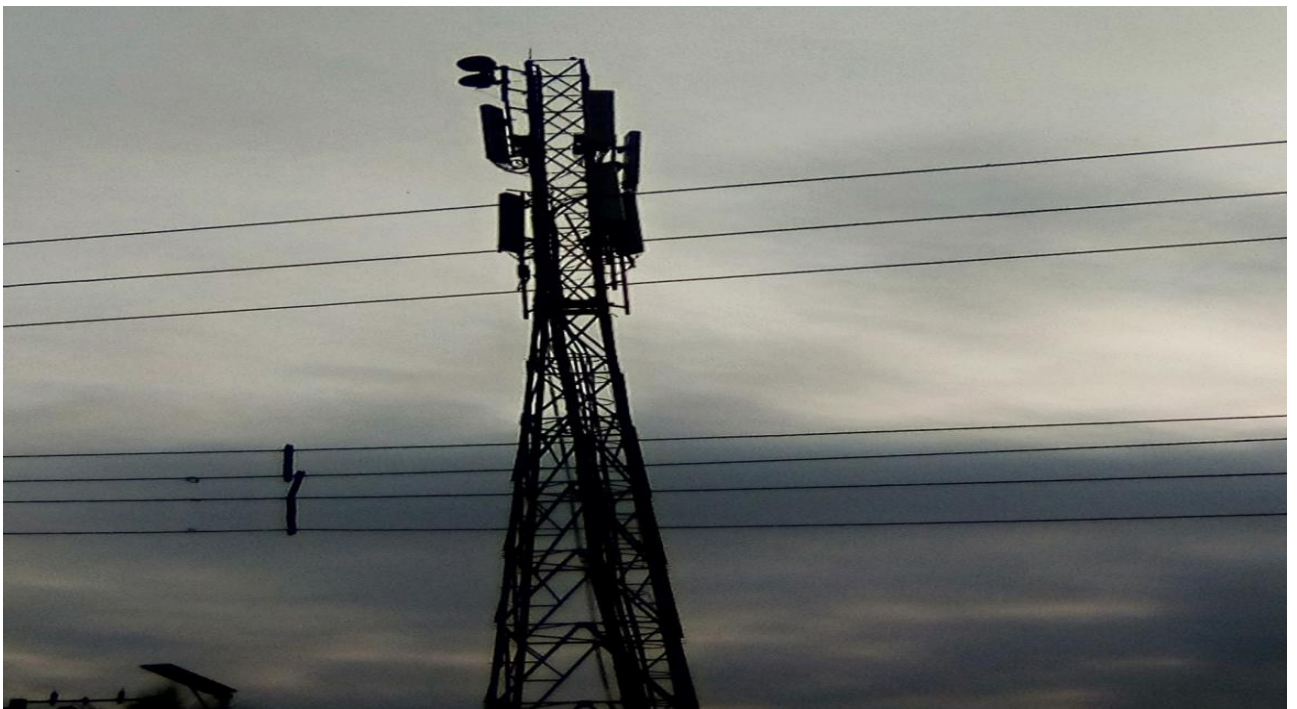
Figure 2.1: A telecommunication mast in Uyo
