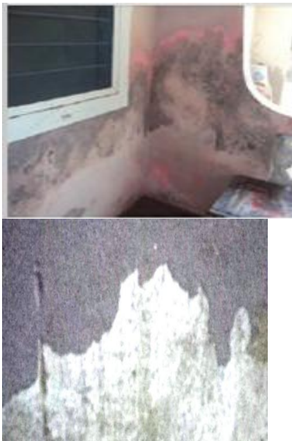
a) Stain in the horizontal band; b) Water run marks on windows; c) flaking of paint Figure 1: Affected areas of building identified during visual inspection
