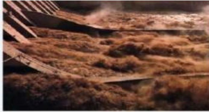
**Figure 5: Using the operation of storing clean water and discharging muddy flow to mitigate reservoir sedimentation (Adapted from Pramoda, 2017)**
